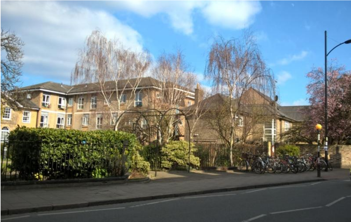
Fig 2: Ditchburn Place from Mill Road, with a view of Burmaside House at the SE corner of the site.
