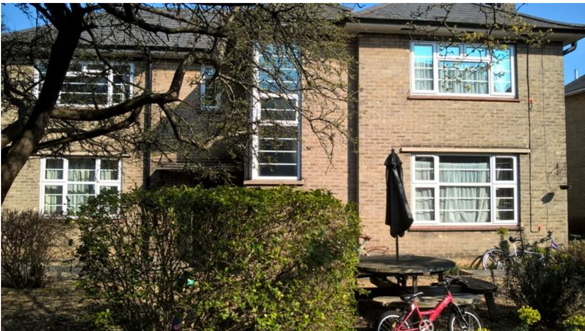
Fig 5: Burmaside House, front. Note tall 'modernist' corner window, which "echoes" the tall ribbon windows of the Nurses' Home, in miniature.
