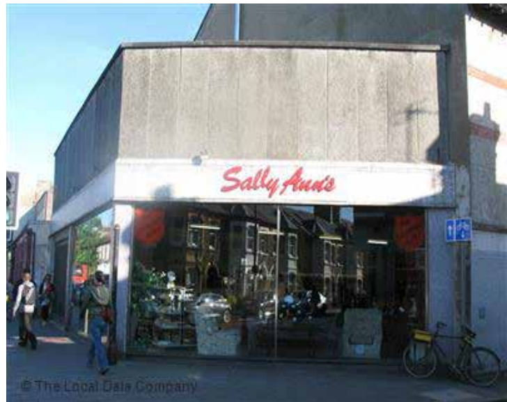
Image courtesy of the Local Data Company
